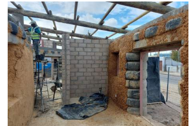
One of the internal walls made from upcycled Polyurethane film set waste
