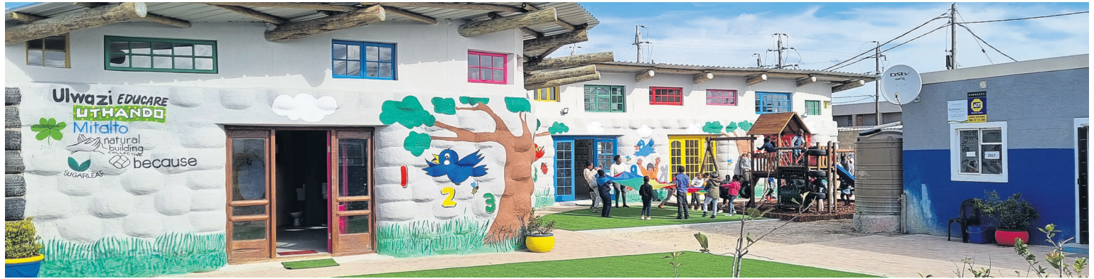
Ulwazi Educare, constructed by Natural Building Collective, is built from tyres, plastic bottles filled with rubbish (eco bricks), polyurethane film set waste blocks and recycled materials. PHOTO: SUPPLIED
