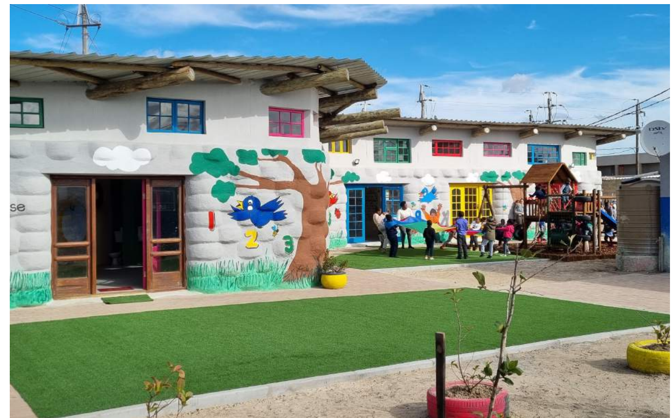
Ulwazi EduCare Centre constructed out of tyres and plastic bottles
